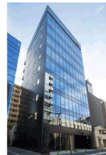
S-GATE FIT八丁堀
